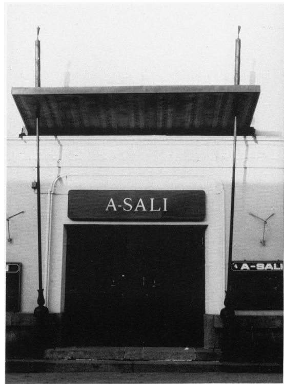
30 Workers' Club, entrance canopy.
